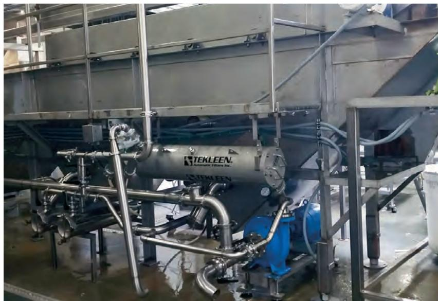
A self-cleaning Tekleen filter unit installed beneath the washing flume
