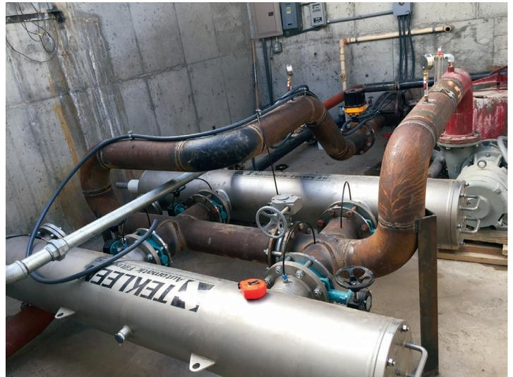
*Tekleen filters 1 and 2 installed in the 1000 Springs Resort pump room.*
