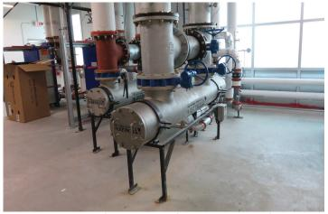
Vision Extrusion Plastics, Vaughan, ON Canada Chilled Water: 2x ABW8-P, 750 gpm , 45 psi, 100µ
