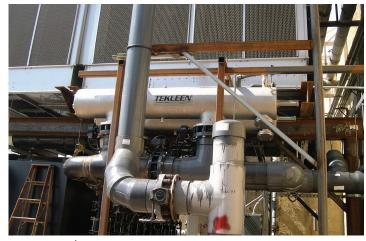
Captive Plastics, Piscataway NJ Cooling Tower: 2 x ABW12-P, 1,100 gpm, 100µ
