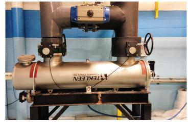
Orbis Plastic Molding Sta Fe, Silao Mexico Process Wwater: ABW6-LP, 600 gpm, 45 psi, 100 µ
